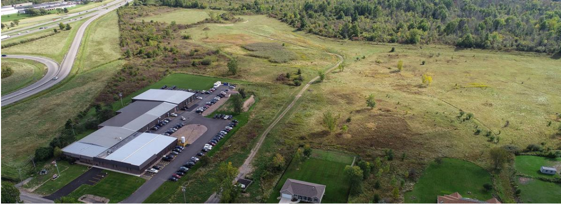
2780 Long Road in Grand Island, where Acquest Development seeks to build a 1.1 million-square-foot warehouse, is shown in his file aerial photo. (Derek Gee/Buffalo News)
